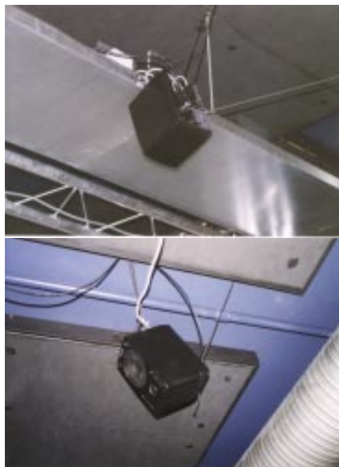
Figure 51: Loudspeakers in the ceiling. Note the two slightly differing ways of mounting them.
