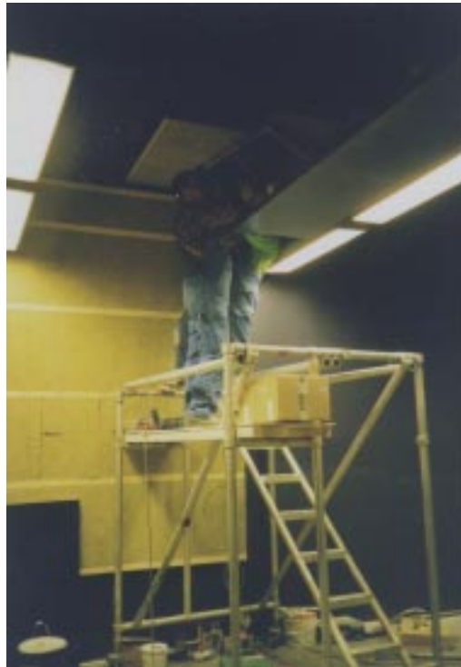
Figure 40: Installing the acoustic panels inside the Cave room.
