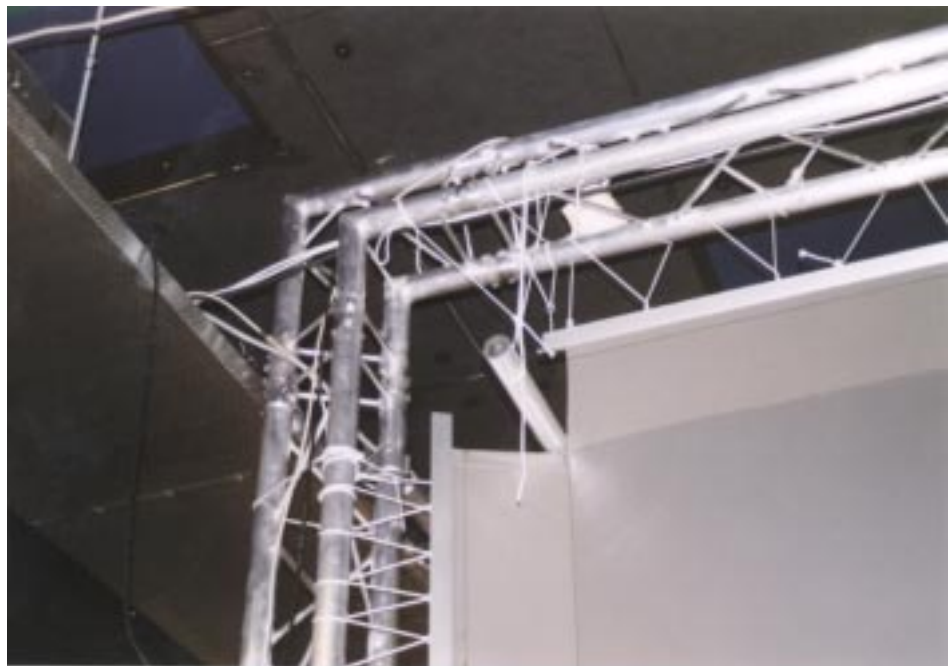
Figure 48: The top left corner. Notice how the vertical and horizontal support bars are attached to the screen itself.
