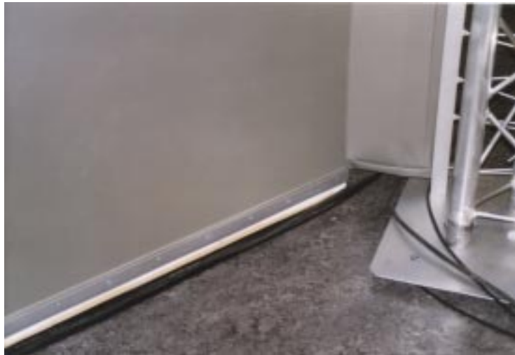
Figure 49: Detail of the front left corner from the outside.
