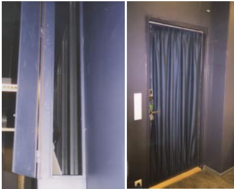
Figure 41: Covered windows (left) and the door (right).
