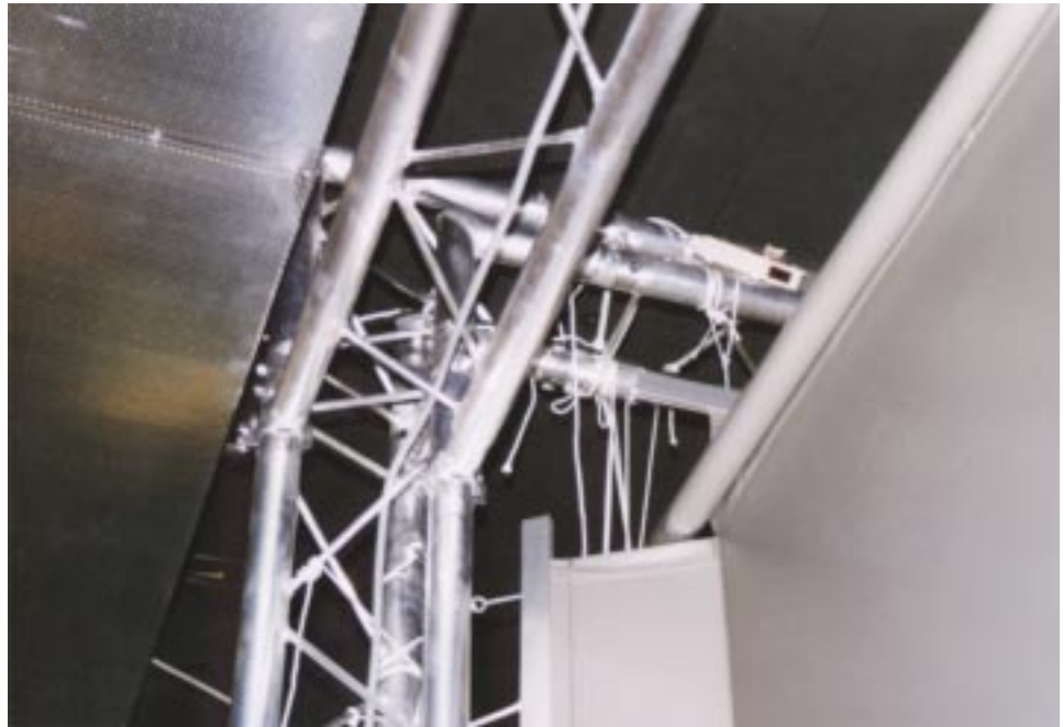
Figure 47: Detail of the front corner. Notice the bar around which the front screen is wrapped.
